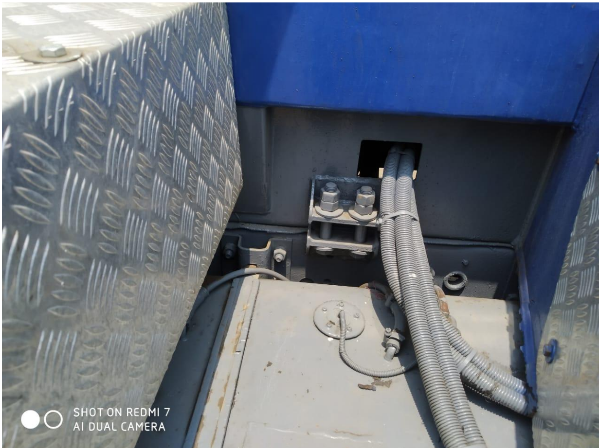
Picture-4 Bolting of chassis of vehicle and beam of Sky lift
